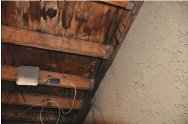
Membrane roof structure below A/C platform. No visual moisture damages nor water stains on plywood and joists detected. Gravel fill is dry.
