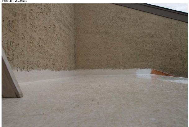
Membrane roof surface below A/C platform also looks fairly new. Ventilation cap in good condition and properly secured.
